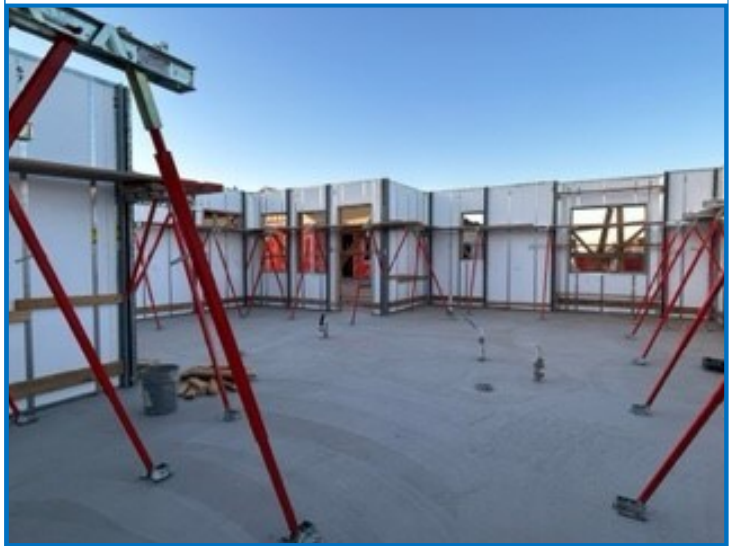
Figure 6. Hercuwall Wall System using SCC ready-mix plants in Arizona regularly produce SCC for the Phoenix Metro area, primarily for high
