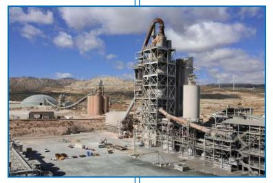
ment. They do this by first grinding all the different materials up very fine, so fine in fact that 80% of all the material will pass a #200 sieve. That means most of the particles are less than 3/1000ths of an inch in diameter! Of the materials required to make portland cement, limestone or calcium carbonate (CaCO<sub>3</sub>) constitutes the largest percentage at about 80%, about 20 to 22% made up of silica (SiO<sub>2</sub>, which
