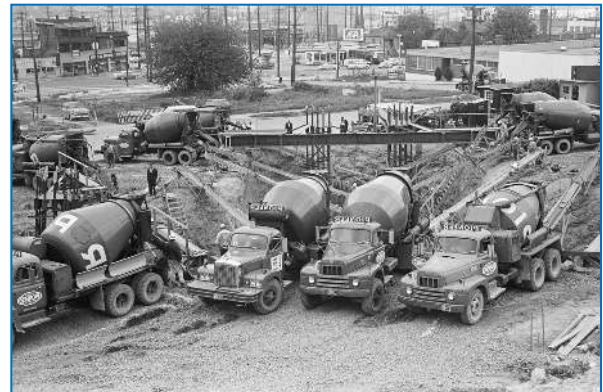
Pioneer Sand & Gravel trucks pouring concrete for the Space Needle in Seattle, WA. c.1961
